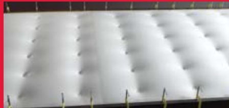
RhinoBond spreads wind load across the roof
