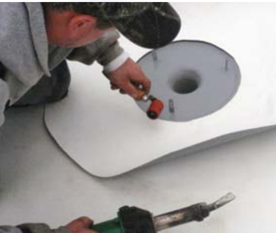
Hercules style retrodrains are available with PVC and TPO coated flange for direct membrane attachment.
