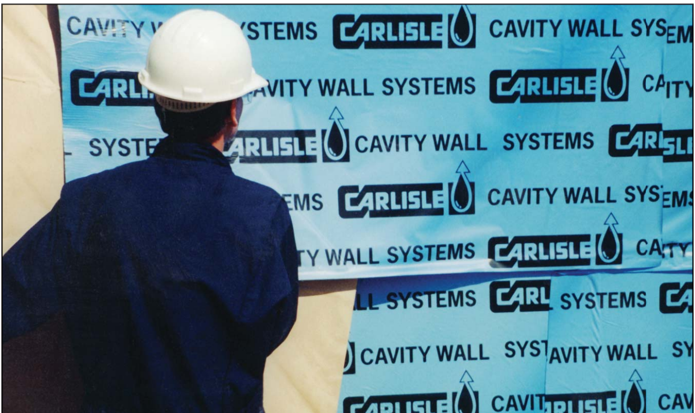
CCW-705 Air & Vapor Barrier Application
