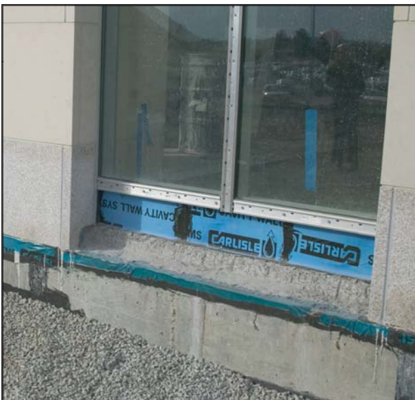
CCW-705 Air & Vapor Barrier Strips Application
