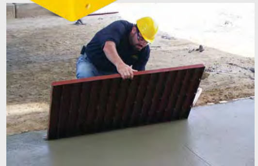
Panel is aligned with bottom edge of curb ramp. Rotate panel down into the wet concrete.
