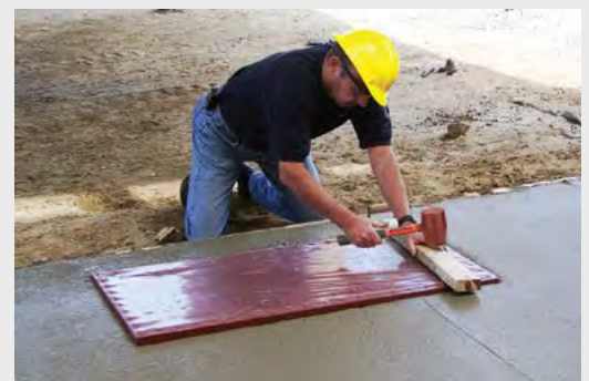
Press panel into wet concrete until top surface is even with surrounding concrete. A rubber mallet and scrap lumber can be used to set panel to proper depth and remove any air pockets under the panel.
