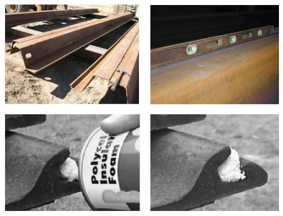
Use urethane foam or similar material to dam ends of interlock.
