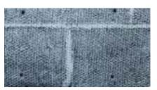
2) The scratch coat is applied with complete embedment of the selffurred lath in the plaster.
