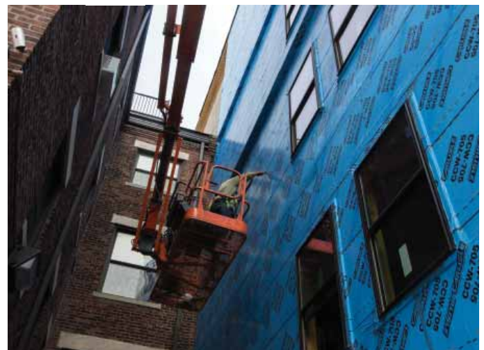
CCW-705 Air & Vapor Barrier Strips Application.
