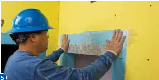
5 Apply LiquiFiber onto wet membrane.
