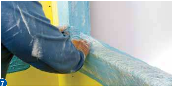
7 Fold LiquiFiber into rough openings and corners. Set tightly in corners with putty knife or similar tool – no bridging.
