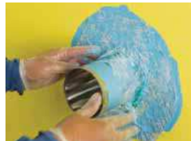
Pipes and Other Through Wall Penetrations
