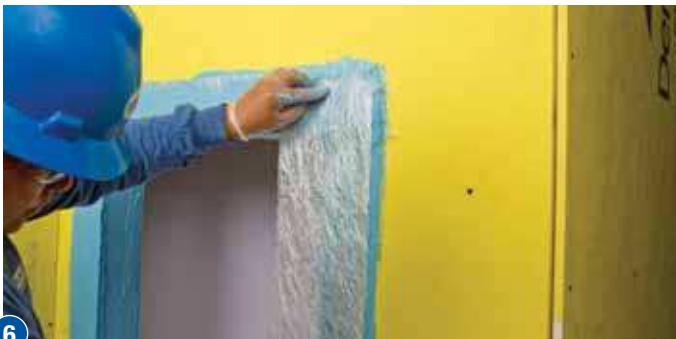
6 Ensure that LiquiFiber overlaps neighboring pieces by at least 2".
