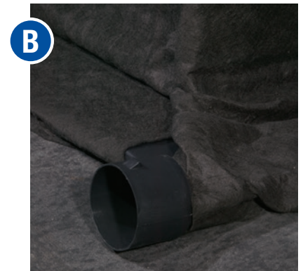
6" Endout Connector covered with fabric
