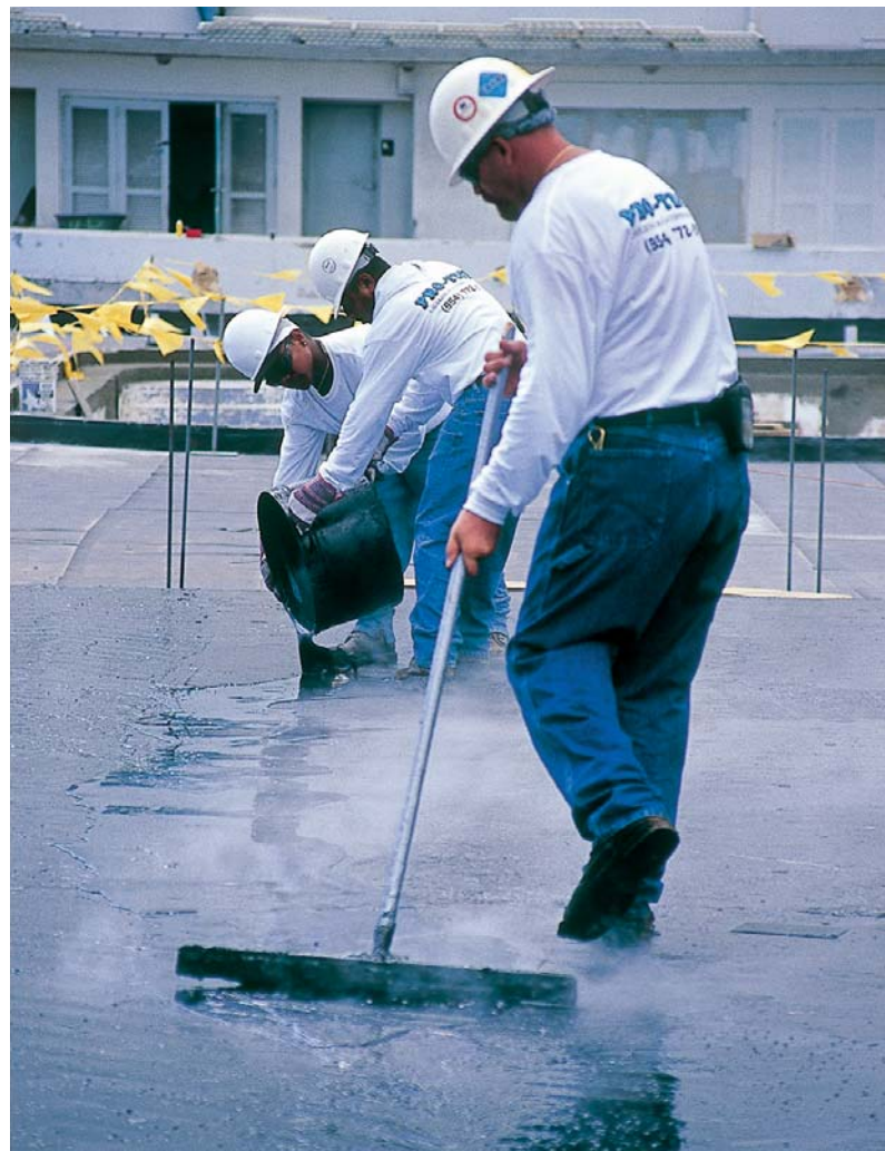
Above: CCW-500R Waterproofing System is one of the essential components available for CCW Green Roofs.
