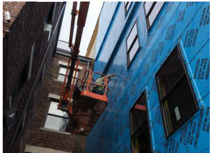
CCW-705 Air & Vapor Barrier Strips Application.
