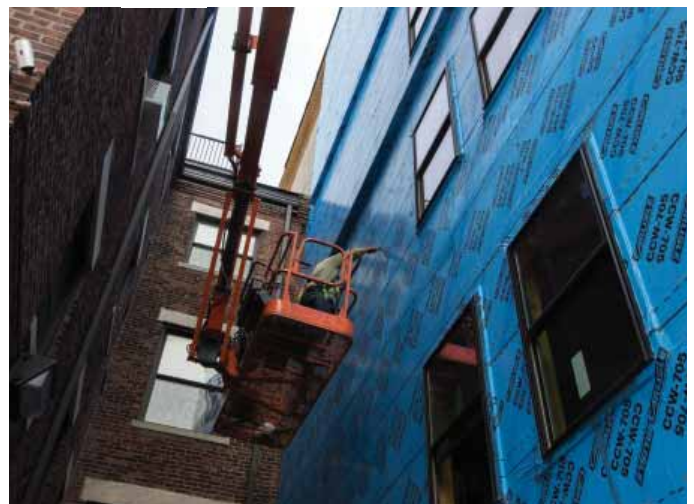
CCW-705 Air & Vapor Barrier Strips Application.
