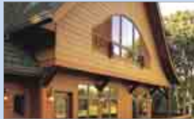
Fiber Cement Siding
