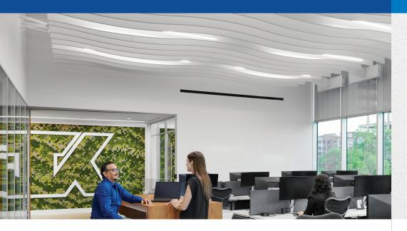
Vertically installed, unframed baffles provide sound absorption and design flexibility.
