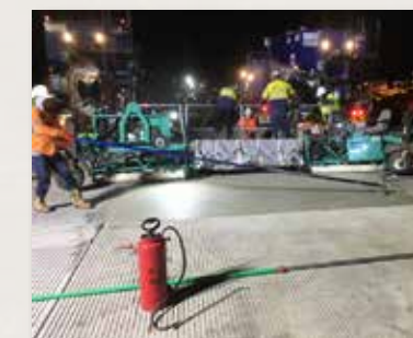
1:30-2:00 Concrete Finishing
