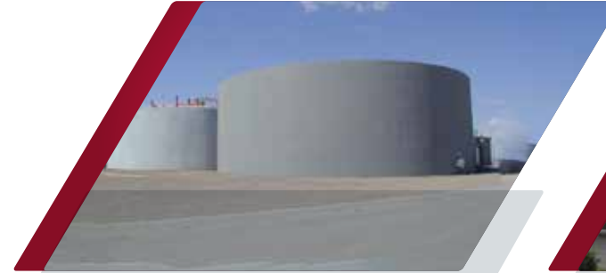
WATER/WASTE CONTAINMENT Treatment, Storage, Containment
