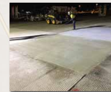
2:00-5:00 Concrete Pavement Reopened
