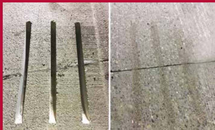
Dowel Bar Retrofit on I-5, Washington
