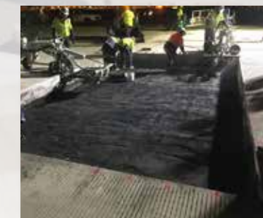
0:45-1:00 Dowel Installation
