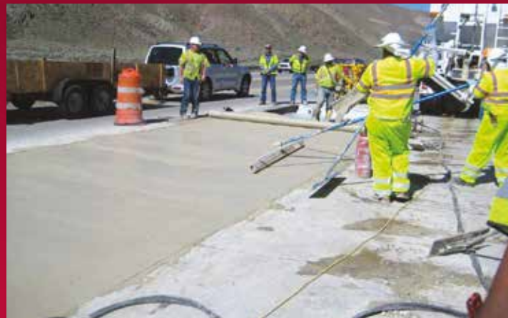
Emergency Panel Replacement on I-80, Nevada
