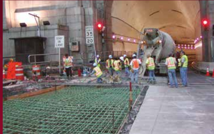
Panel Replacement at the Lincoln Tunnel, New York City
