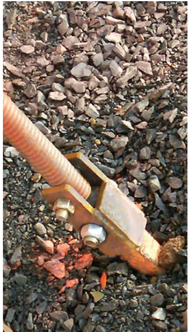
INCORRECT Brace-to-HGA Connection
