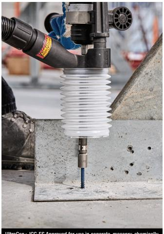
UltraCon+ ICC-ES Approved for use in concrete, masonry, chemically treated lumber and wood-to-wood applications.
