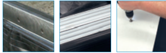
SJS-FP installation consists of the two sub-assemblies which make up the system. The mounting leg assembly and integral waterproof sidesheets are installed onto the structural slab and integrated with the deck waterproofing system. The watertight, precompressed SJS assembly is installed between the rails of the mounting leg assembly and then capped with an aluminum or stainless steel coverplate.
