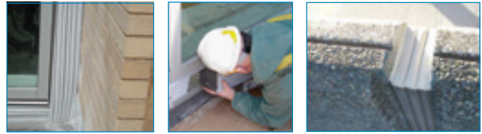
Seismic Colorseal-DS seals interior and exterior sides of curtain wall joints in a single installation step. Each side can have its own color to match interior and exterior color schemes. For parapets it can provide a top, front, and back sealed surface addressing all three exposed planes.
