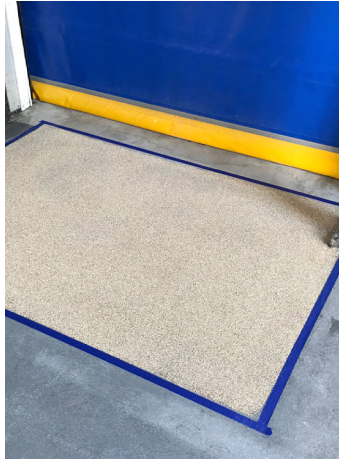
Broadcast calcined Bauxite applied over epoxy coating and RSR Easy Mix™ resulting in an R14 non-slip surface.
