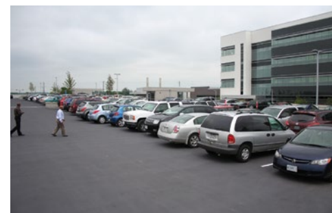
(Above and Far Left) Research In Motion, the makers of Blackberry cell phones, converted their parking lot to cool pavement that qualified for LEED® points using StreetBond® SB150 Pavement Coating with SR Slate Colorant. The SR Colorant uses special technology to provide solar reflectivity even though it is a darker slate color.
