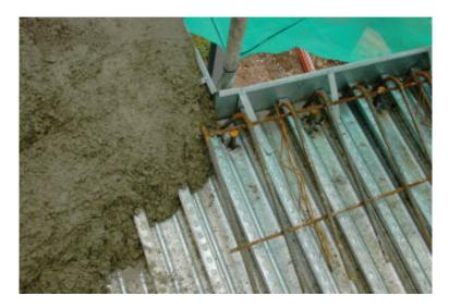
STRUX <sup>®</sup>90/40 fiber as marketed by GCP Applied Technologies is classified by Underwriters Laboratories Inc. for use as an alternative, or in addition to, the welded wire fabric in 1, 11/2 and 2 hr floor-ceiling D700, F700, D800, F800, D900 and F900 (except 909) Series Designs. Fibers to be added to the concrete mix at maximum addition rate of 5 lbs/yd<sup>3</sup> (3.0 kg/m<sup>3</sup>).
