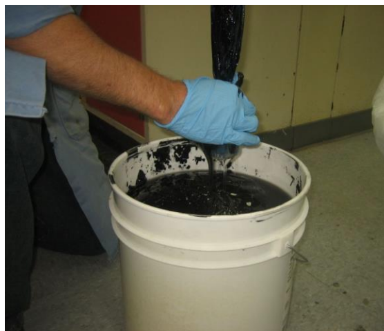
Wring excess liquid from blue liner
