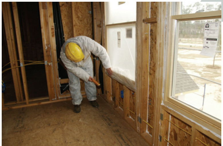
Figure 10: Sealing the windows
