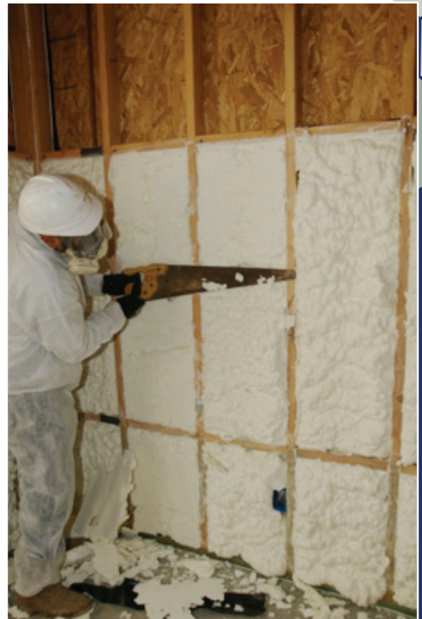
Figure 15: Contractor trimming foam
