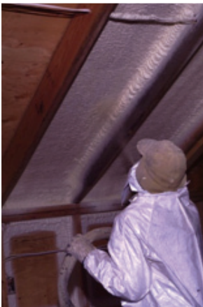
Figure 16: Maintain average thickness throughout
