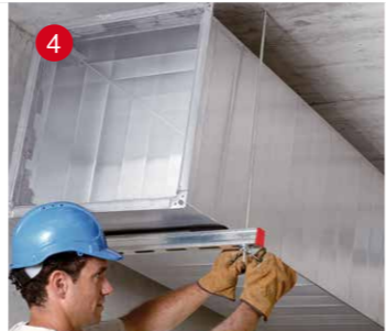
4 Mechanical & electrical, HVAC
