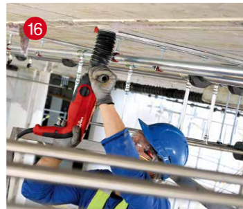
16 Post-installed anchors
