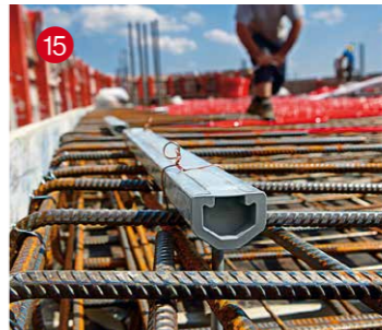
15 Cast-in anchors
