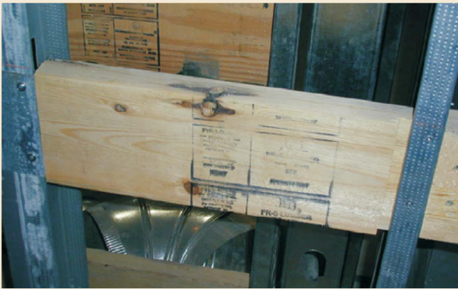
PyroGuard™ is frequently used as blocking in the walls of Type I and II construction. Cleveland, OH.
