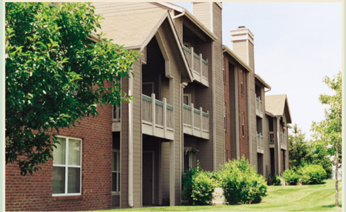
Sprinklers may be eliminated from balconies constructed of ExteriorFireX™. Kansas City, MO.
