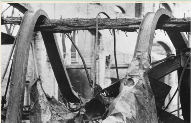
In 1953, a fire in a casein glue factory demonstrated the superior fire-endurance of untreated wood over steel.
