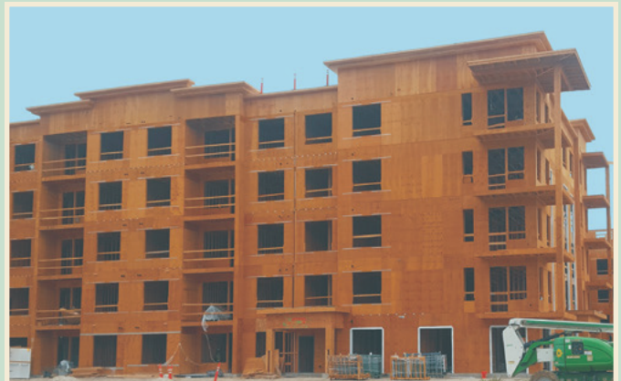
Type III: UL Design No. V314 used PyroGuard™ for the 2-hour bearing exterior walls in Draper, UT.
