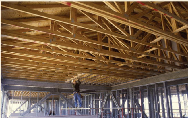
PyroGuard™ roof systems can eliminate sprinklers in concealed spaces of any type of construction.
