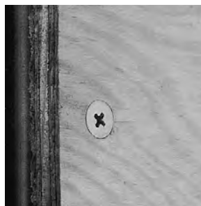
Plywood to steel or wood studs
