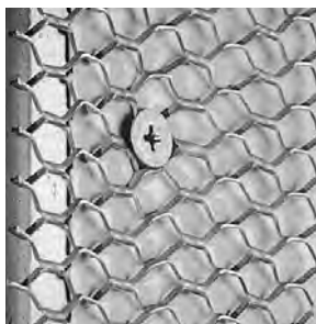
Wire lath to steel or wood studs
