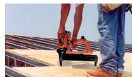
Plywood attachment—using TrakFast plywood to steel pin
