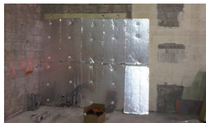
Interior walls on concrete block
