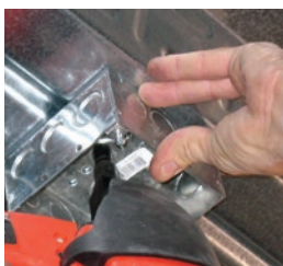
M100 fastener used to attach a junction box
