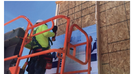
Behind cladding over wood stud walls
