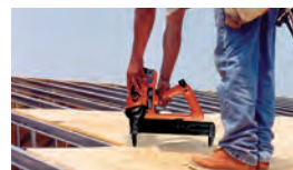
Plywood attachment—using TrakFast plywood to steel pin
