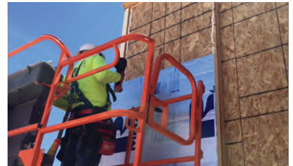
Behind cladding over wood stud walls
