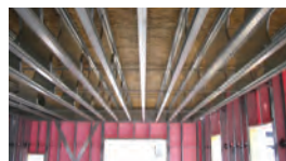
OSB and plywood to ISPAN joists
