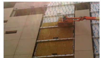
Behind cladding over concrete block walls
