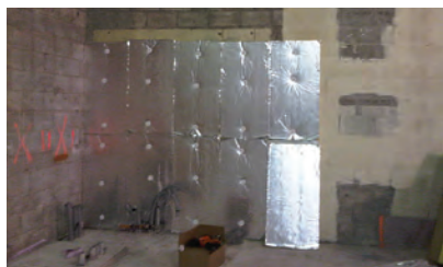
Interior walls on concrete block
