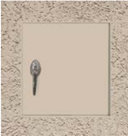
Example of XPEA Installed in Stucco Wall
