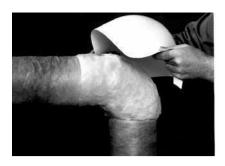
1. Position the Zeston PVC fitting cover over the insulated fitting.
