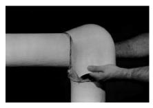
Place the fitting cover over the insulation, lapping the mastic-covered edge over the other side of the throat seam.
