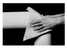
2. Place the pre-cut fiber glass insert around the fitting, positioning the points of the insert on the inside radius of the elbow. For applications with temperatures below 45°F (7°C) or above 250°F (121°C), additional layers of insulation may be required.\* In such cases, the first layer is secured by wrapping with fiber glass yarn.
