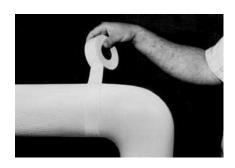
As an option, apply color-matched, pressure-sensitive Z-Tape to the butt joints for a more attractive appearance.
