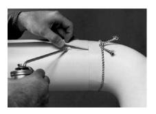
4. Overlap the jacketing on itself (approximately 1½" to 2" [38 mm to 51 mm]) and apply a bead of adhesive along the entire length of the longitudinal lap. Place elastic cords or PVC tape around the jacketing.
