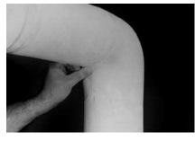
After the fitting cover is in position, push the tacks into the overlapping throat seam. No further fastening is required.
