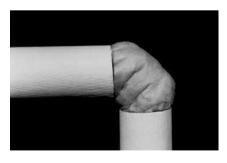
3. Butt the ends of the fiber glass insert against the ends of the pipe covering. Tuck and fold the insulation so that it covers all bare surfaces. Keep the fiber glass fluffed up to the thickness of the adjacent pipe insulation to assure maximum thermal efficiency.
