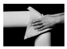
2. Position, tuck, and fold the fiber glass insulation insert as described below in steps 2 and 3 for hot systems.
