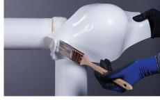
**5**. Apply the mastic along the inside of the fitting cover throat overlap seam. Pressure-sensitive Z-Tape or serrated tacks may also be used.
