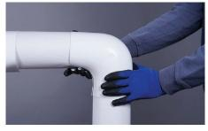
**5**. After the fitting cover is in position, push the tacks into the overlapping throat seam. No further fastening is required.
