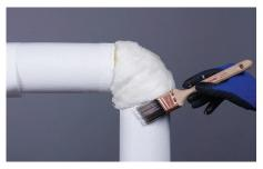
**4**. Apply a vapor barrier mastic around the edges of the adjoining pipe insulation.
