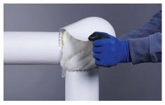
**1**. Position the Zeston PVC fitting cover over the insulated fitting.
