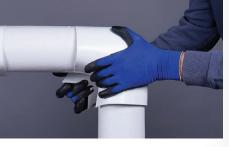
**6**. Place the fitting cover over the insulation, lapping the mastic-covered edge over the other side of the throat seam.
