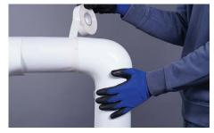
7. Apply Z-Tape over the circumferential joints. The tape should extend over the adjacent pipe insulation and overlap itself by at least 2" (51 mm) on the downward side of the lap. The tape provides securement, an attractive appearance, and completes the vapor seal.
