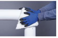
**2**. Place the pre-cut fiber glass insert around the fitting, positioning the points of the insert on the inside radius of the elbow. For applications with temperatures below 45°F (7°C) or above 250°F (121°C), additional layers of insulation may be required.\* In such cases, the first layer is secured by wrapping with fiber glass yarn.
