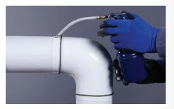
**3.** After the fitting cover has cured at least 10 minutes, run a bead of adhesive along its circumferential edge. Overlap the fitting cover (by approximately 1" [25 mm]) with a section of Zeston PVC jacketing and secure the circumferential joint with an elastic cord. The cord may be removed after approximately 10 minutes.
