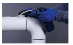
**4**. Overlap the jacketing on itself (approximately 1½" to 2" [38 mm to 51 mm]) and apply a bead of adhesive along the entire length of the longitudinal lap. Place elastic cords or PVC tape around the jacketing.
