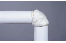
**3**. Butt the ends of the fiber glass insert against the ends of the pipe covering. Tuck and fold the insulation so that it covers all bare surfaces. Keep the fiber glass fluffed up to the thickness of the adjacent pipe insulation to assure maximum thermal efficiency.
