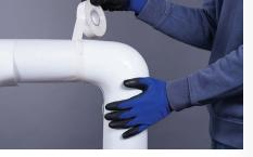
**6**. As an option, apply color-matched, pressure-sensitive Z-Tape to the butt joints for a more attractive appearance.
