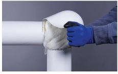
**4**. Insert two stainless steel serrated tacks approximately ¼" (6 mm) from one of the lap edges of the fitting cover. Then snap the cover in place over the fiber glass insulation.
