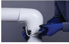
**2**. Using a standard applicator gun or squeeze bottle, apply a bead of Perma-Weld adhesive along the throat overlap of the fitting cover. Snap the fitting cover into place and secure with elastic cord or PVC tape. Always feather the adhesive along the seam.
