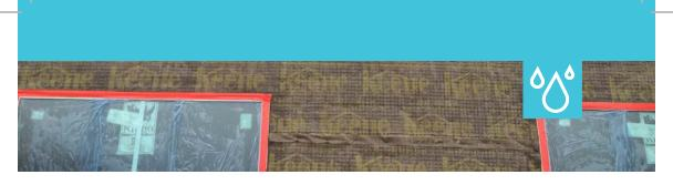
Driwall<sup>™</sup> Rainscreen provides an airspace for any incidental moisture penetration that gets behind the stone, which occurs due to wind driven rain. Driwall<sup>™</sup> Rainscreen allows for moisture to drain to the exterior.
