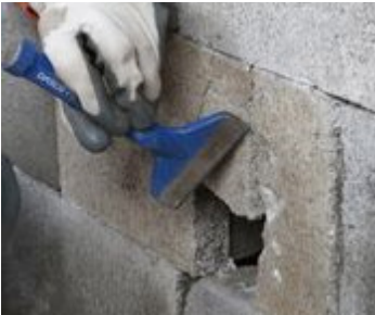
Prepare the surface
