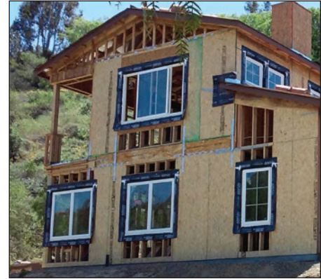
MFM waterproofing membranes are self-sealing around fasteners to maintain a waterproof seal.
