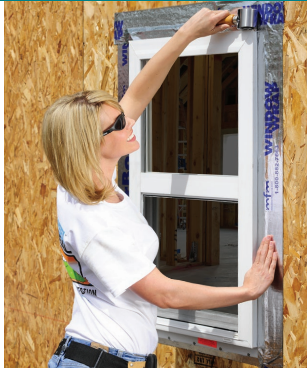
The WindowWrap® family of products are self-adhering, self-sealing waterproofing tapes designed for use around windows, doors, building seams and in general construction.
