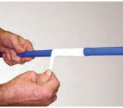
3. When the joint is complete and cool, replace the plastic coat and wrap the joint to give continuity of protection
