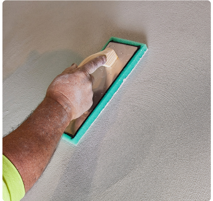
Finish (second) coat (Smooth or Texture Finish)
