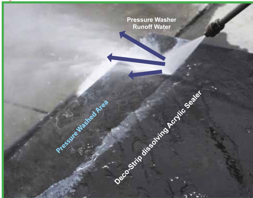
CORRECT PRESSURE WASHING SPRAY METHOD
