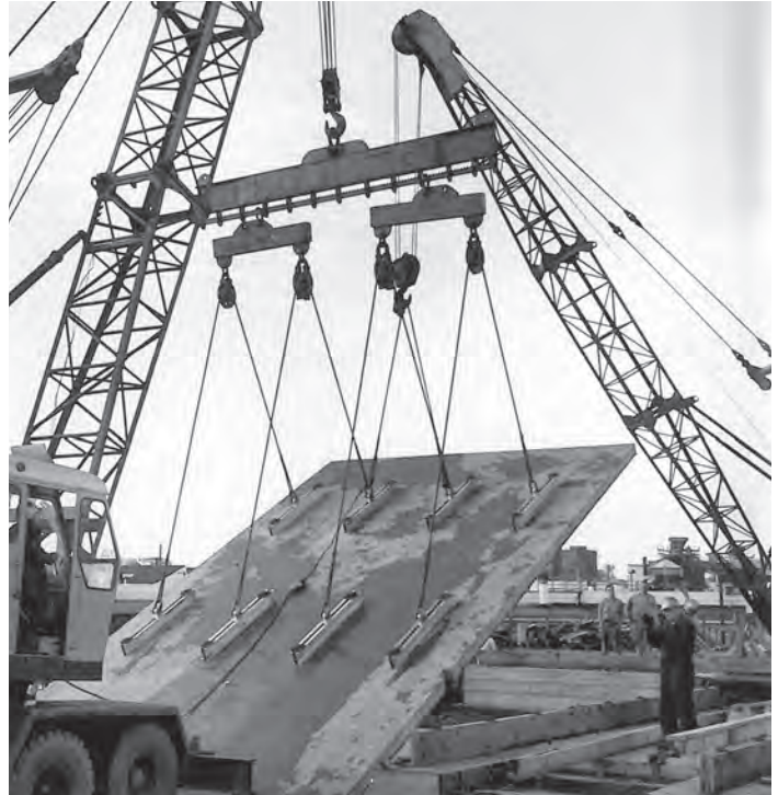
NOX-CRETE BONDBREAKER USED ON CIRCA 1964 TILT-UP PROJECT
