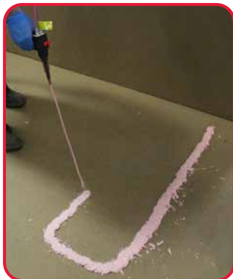
Bead Applied 6" from Surface Using Extension tube
