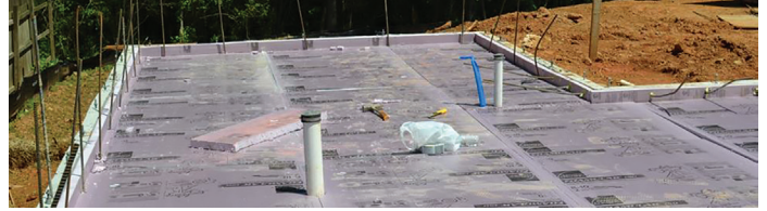
Boards should be installed tightly together.
