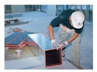
elbows, tees, offsets and other system elements can quickly and easily be fabricated at the shop or on the job and assembled into a complete air transmission system.
