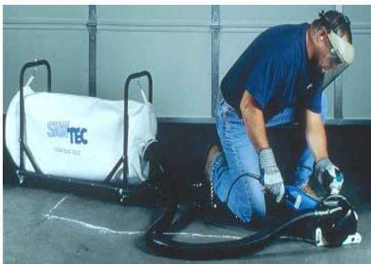
Photo #13 - Diamond Grinding
