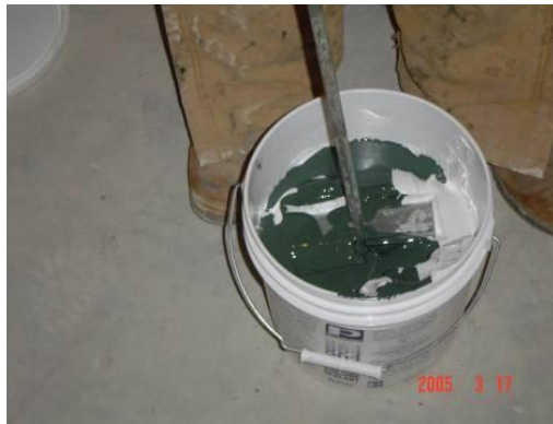
Photo #15 – Sealant Mixing in Process
