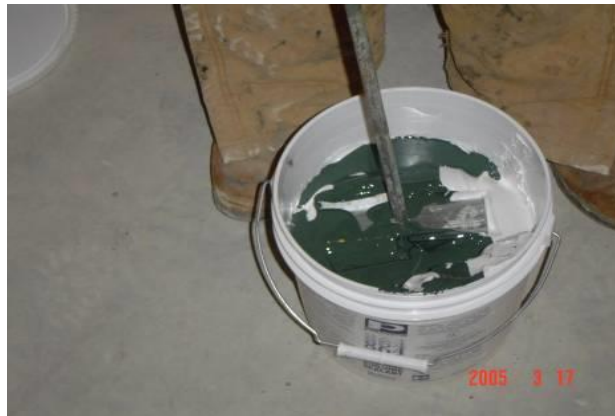
Picture #15: Sealant Mixing in Process
