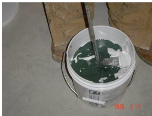
Photo #15 – Sealant Mixing in Process
