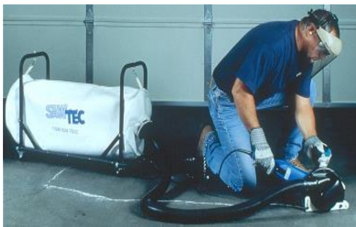
Picture #13: Diamond Grinding
