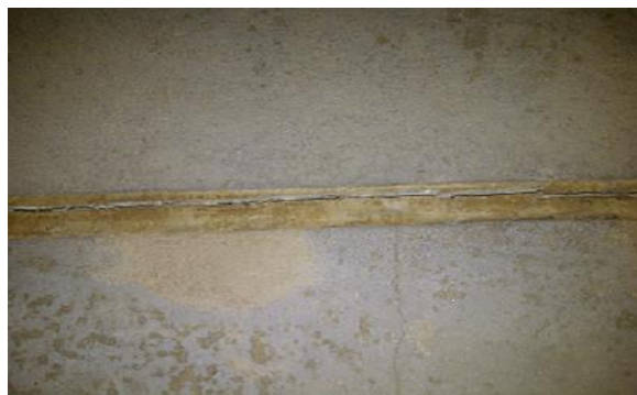
Picture #10: Cohesive Failure
