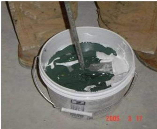
Picture #4: Multi-component sealant mixing procedure
