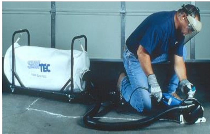
Picture #13: Diamond Grinding
