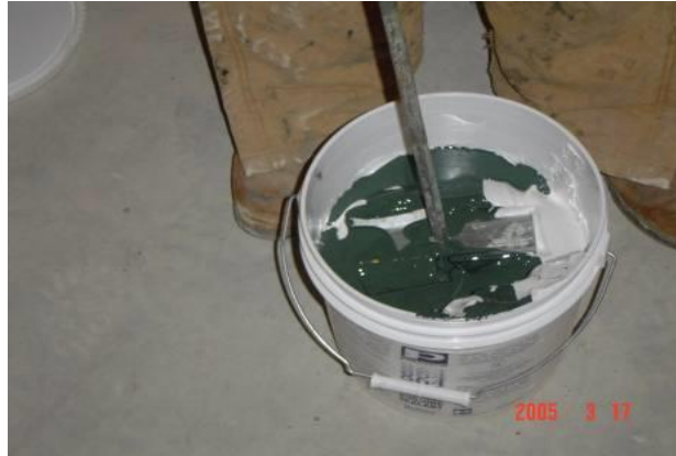
Picture #15: Sealant Mixing in Process
