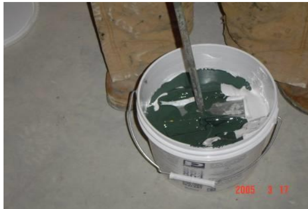
Picture #15: Sealant Mixing in Process
