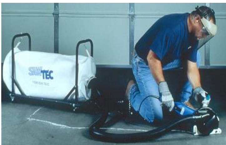
Picture #13: Diamond Grinding
