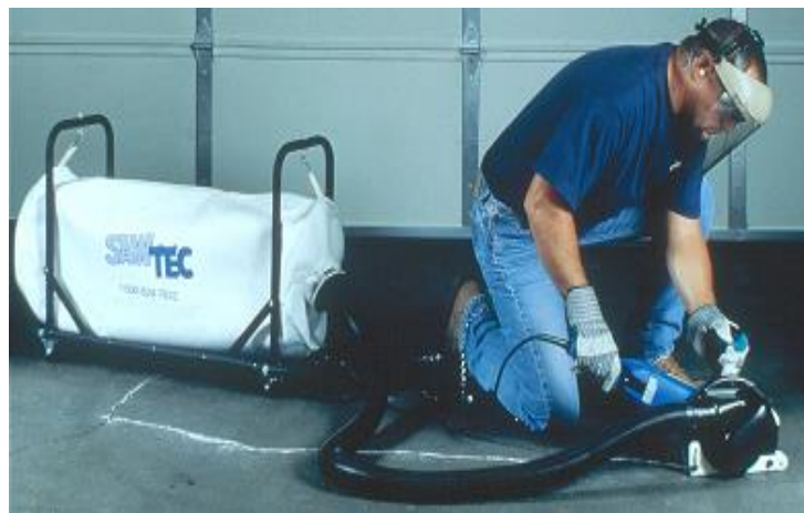
Picture #13: Diamond Grinding
