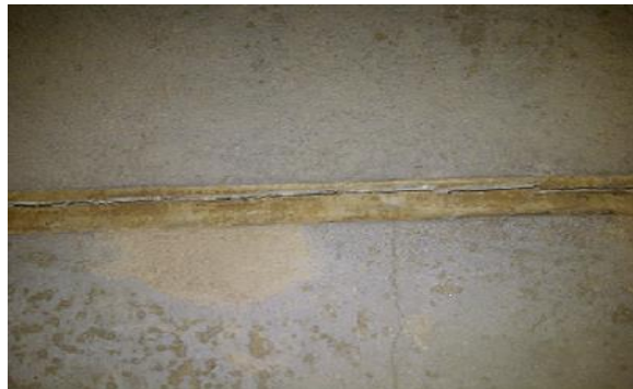
Picture #10: Cohesive Failure
